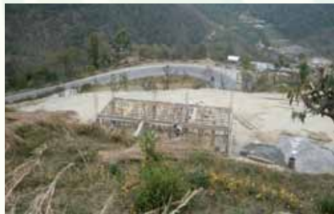
Fulbari Resource Centre -Under construction
